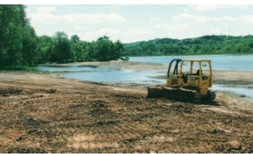
Bulldozer removing contaminated sediment from Nahant marsh. USFWS photo.
