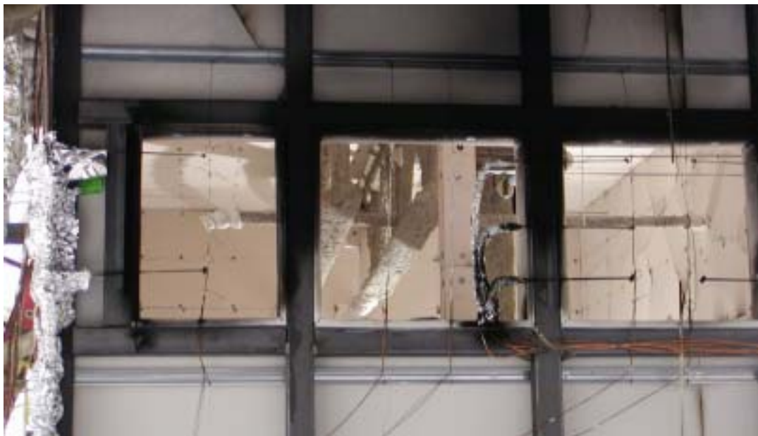
Figure 4. View of compartment from air exhaust outlet prior to the start of test 6. The foreground shows instrumentation for characterizing the air flow at the outlet.
