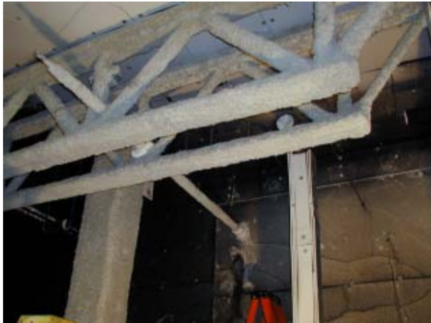
Figure 2. Insulated steel components in place prior to Test 5. In the foreground are two steel trusses and a steel rod, supported across the lower chord panel points, positioned near the ceiling above the fire pan. The steel column is located between the air inlet and the fire pan. The specimens are similar in geometry but not exact replicates of those in the WTC towers. The tests are designed to validate models to analyze heat flux and temperatures models.
