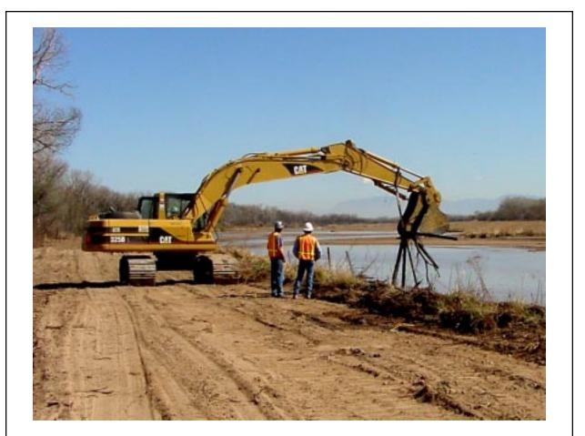
Fig. 17: Los Lunas, west bank. The first day of jetty jack removal, Apr. 9, 2002. Bankline jacks are the first to be removed. The job of removing 1,355 jacks is expected to take one to several months. Photo by Mark Horner, U.S. Army Corps of Engineers.
