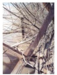
Fig. 14: The MRGCD wants riverbank jacks to stay in place for levee protection
