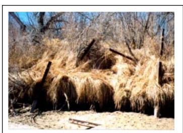
Fig. 16: In the Rio Grande facing west at the Los Lunas restoration site, west bank. Note the buried jack in the foreground center bottom. The jetty line in the bank respresents the landward diversion line installed behind the riverward line. Both lines will be removed.
