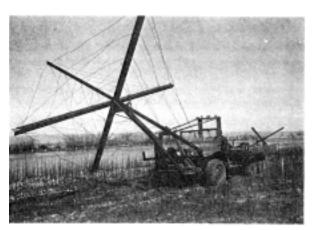
Fig. 4: Jack unit is moved to position in jetty field by a winch controlled lift. Casa Colorada area, Middle Rio Grande Project, NM. Photo:Herman E. Carter, Bureau of Reclamation (Carlson and Enger 1956).
