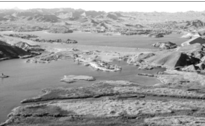
Phase I Safety of Dam activities were completed at Senator Wash Dam, California.
