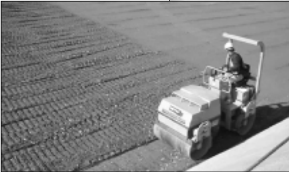
Repair work at Pueblo Dam (inset) and spillway test (right) following completion.
