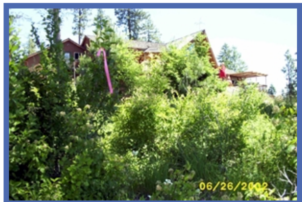
A wildland urban interface home nearly obscured by vegetation.
