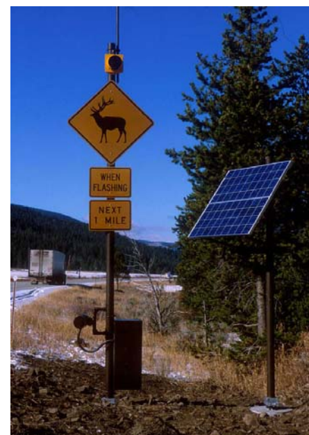
RADS system being tested along a Montana highway.
