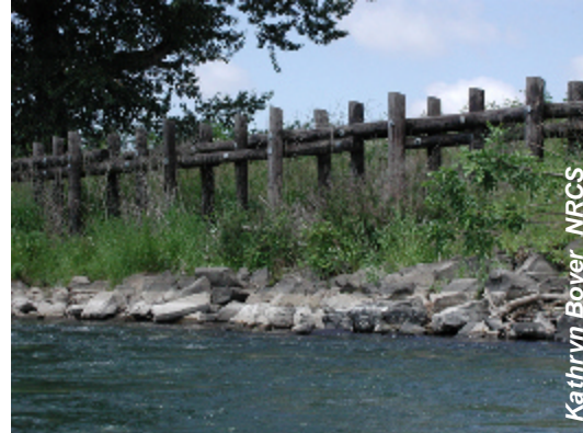
Figure 9. Rock and timber revetment on the Willamette River, Oregon.
