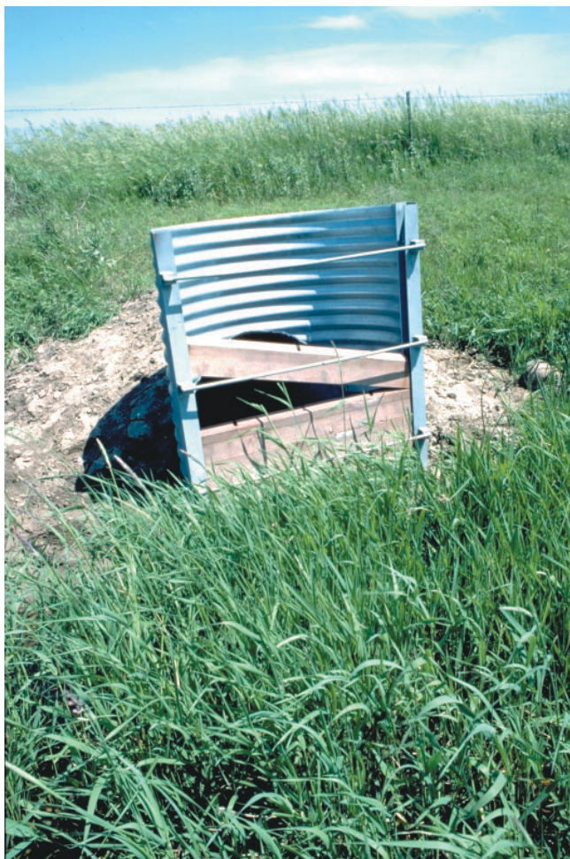
Photo 9-1. Simple controlled drainage devices can be constructed using culvert materials and flashboards that can be added and removed to adjust outflow. (Tim McCabe photo)
