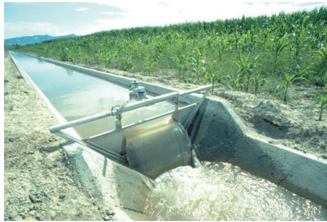
Photo 6-1. On a secondary lateral a water control structure regulates irrigation water delivery for the adjacent cropland. (Tim McCabe photo)
