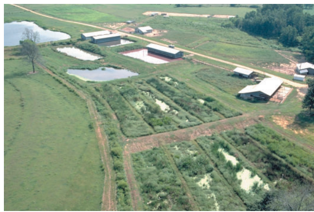
Photo 8-3. In Alabama a constructed wetland is used to filter waste from a hog operation. (Tim McCabe photo)
