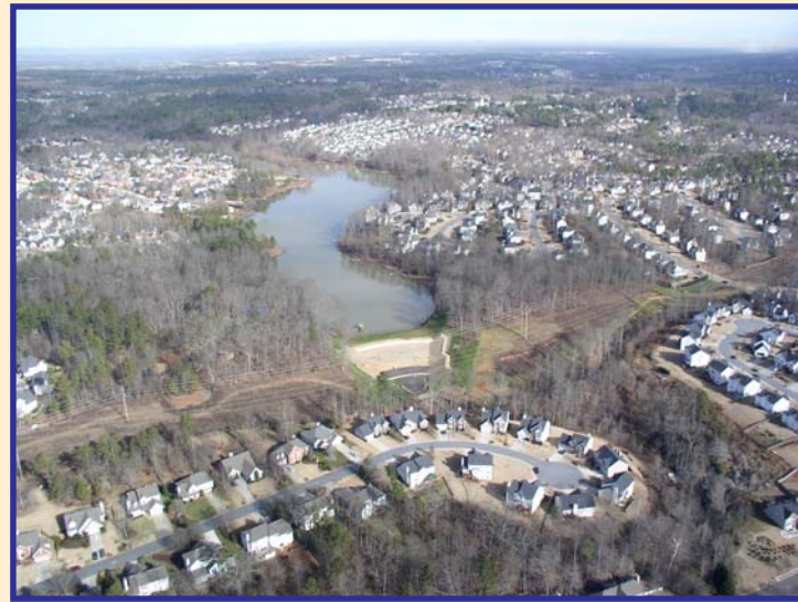
Yellow River Watershed Dam No. 14, Gwinnett County, Georgia. This dam was built in 1968 as a significant hazard dam under the Resources Conservation and Development Program (RC&D). The significant classification was based upon the fact that two state highways were downstream from the dam. Since 1968 the population of the county has increased from 73,000 to 625,000 and urban development has occurred both upstream and downstream from the dam.
