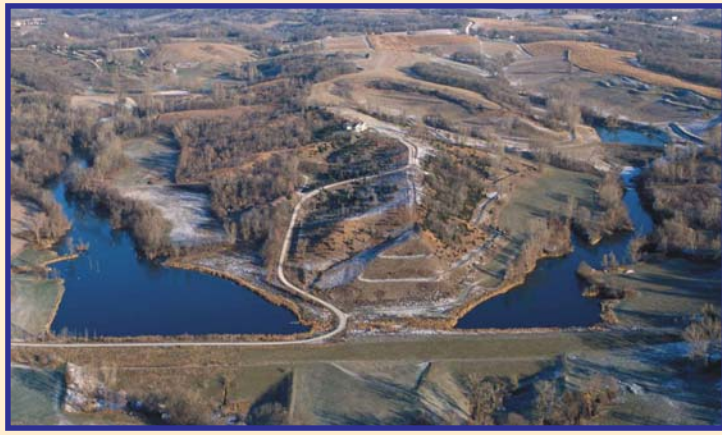
Indian Creek Dam No. 2, West Pottawattamie County, Iowa. This 70-foot high dam was built as a grade stabilization structure on a tributary to Indian Creek. It is one of several dams built upstream from the city of Council Bluffs to control erosion and downstream flooding. The 29-acre lake provides fishing, recreation and wildlife habitat.
