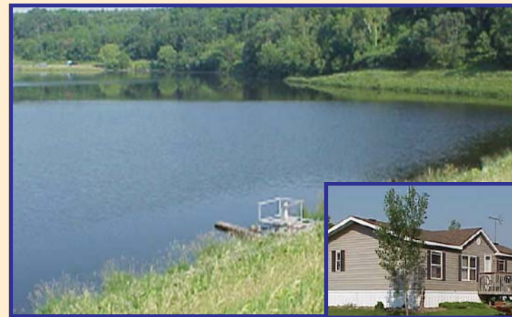
Glenn Hills Dam No. 2, St. Croix County, Wisconsin. This dam was built as a low hazard dam to protect rural agricultural land. After the dam was built in 1972, a home and garage were built downstream from the dam. Rehabilitation funds were used to relocate the home out of the floodplain. Current local zoning now limits residential development downstream from the dam.
