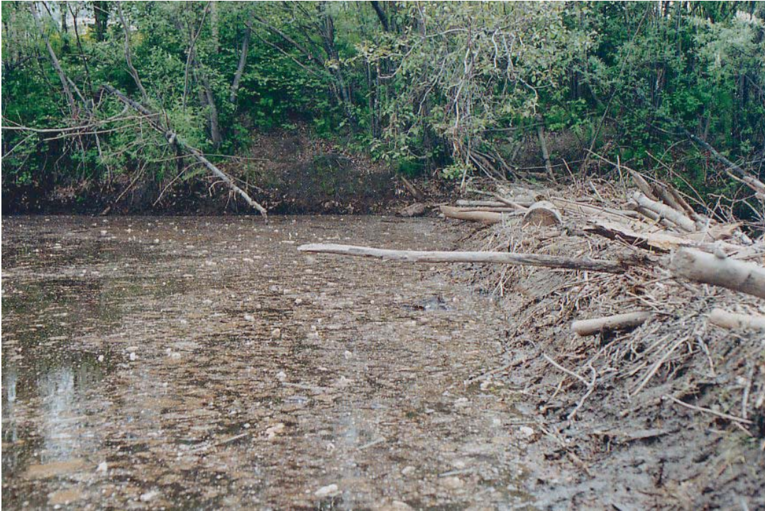
Figure 7. Beaver dam on Noyes Slough, Fairbanks, Alaska. The view is looking across the downstream side of Dam 7 in reach 9, just upstream from Deere Street. This was a likely barrier to fish movement at most streamflow levels during summer 2001.
