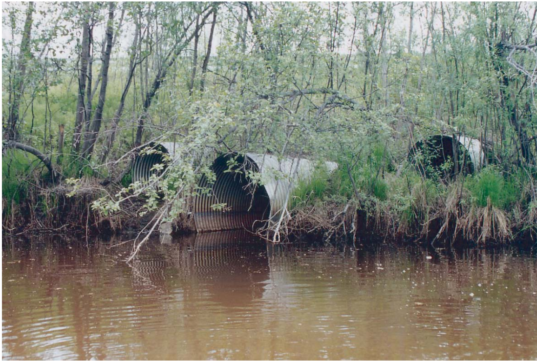
Figure 5. Culvert discharge into Noyes Slough near East College Road, Fairbanks, Alaska.
