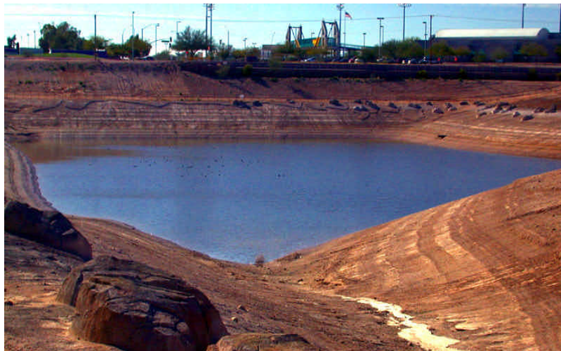
Figure 5. The 7-acre pond at the Tucson Ajo Detention Basin. View is looking to the south; photo was taken January 17, 2003. Tucson Electric Park is in the background.
