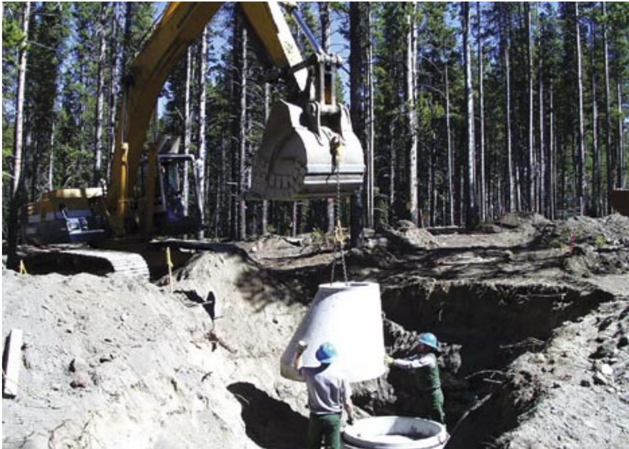
Yellowstone National Park (MT/WY/ID) is replacing failing sewer systems and installing new sewer lines throughout the park to protect park resources and better serve visitors.
