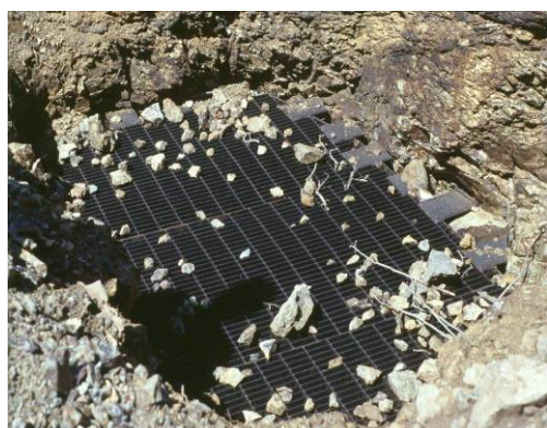
Steel grate closure on vertical opening # 7 in the Orphan Girl project
