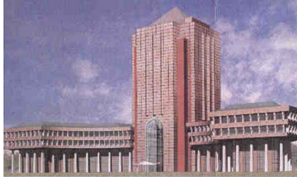
Fig. 1.9. Tokyo University of Technology's Katayanagi Advanced Research Laboratories building, which houses the Bio-nanotechnology Center, Content Technology Center, Advanced IT Center, Creative Lab, Encoding Center, and Bionics Research Center, which is part of the academia-government-industry Collaborative Research Center.
