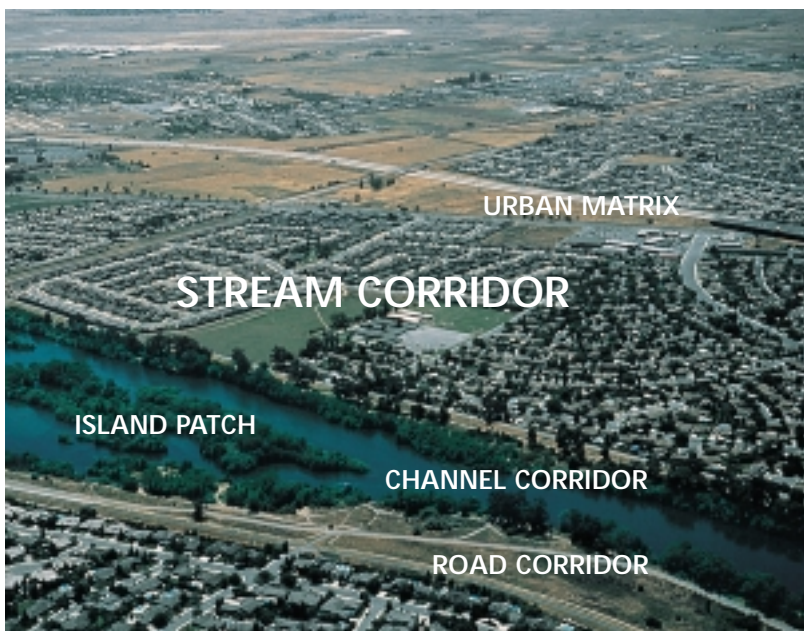
Figure 1.8: Structural elements at a stream corridor scale. Patches, corridors, and matrix are visible within the stream corridor.
