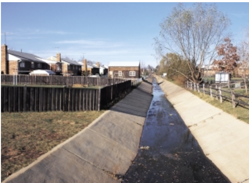
Figure 3.10: Stream channelization. Instream modifications, such as uniform cross section and armoring, result in ecological decline.
