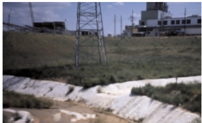
Figure 3.22: Urban stream channel modifications. Channel armoring often prevents streams from accommodating hydrologic changes that result from urbanization.
