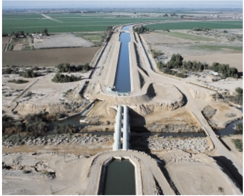
Figure 3.11: Stream diversion. Diversions are built to provide water for numerous purposes, including agriculture, industry, and drinking water supplies.
