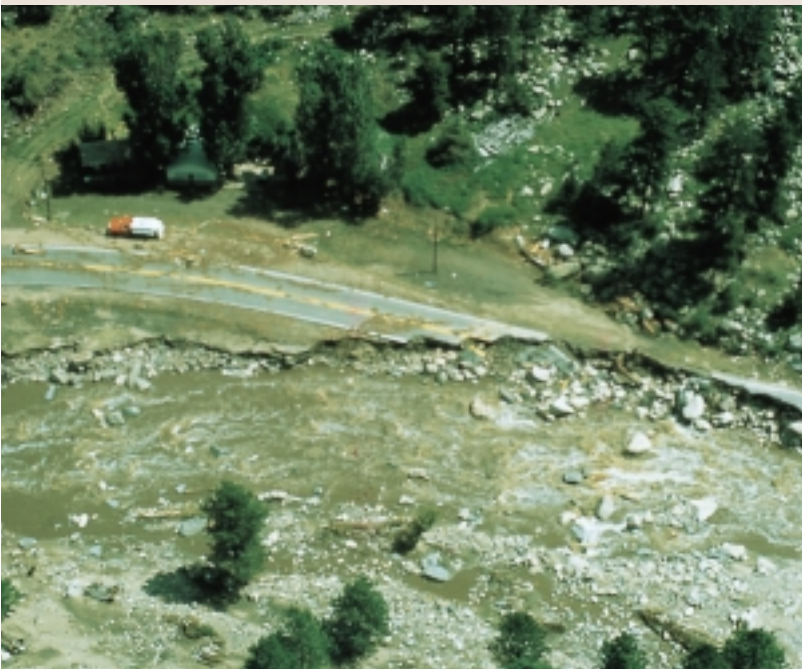
Figure 4.12: Bank erosion. The cause(s) of bank erosion should be identified.
