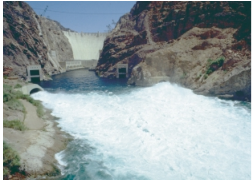
Figure 4.13: Water releases below a dam. Altering the flow regime of river below Hoover Dam altered the stream condition.
