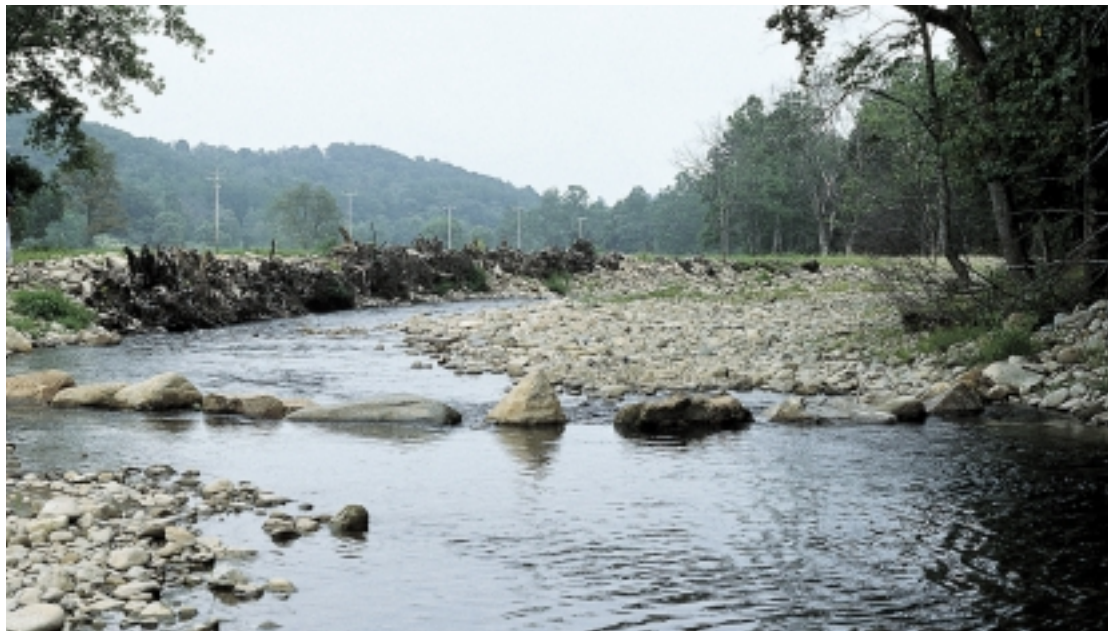
Figure 6.22: Instream modifications. Restoration evaluation may focus on the physical traits of the channel that were intentionally modified during project implementation such as the riffles pictured.
