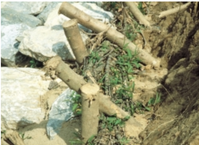
Figure 8.12: Revegetation with the use of deeply planted live cuttings. In arid regions, poles or cuttings of species that sprout readily are often planted to depths that assure contact with moist soil.
