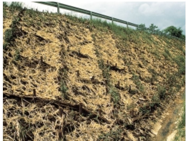
Figure 9.13: A well-mulched site. Mulching is an effective method for improving the final outcome of stream corridor restoration.
