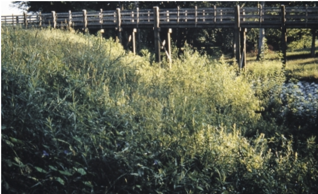
Figure 9.20: Remedial maintenance. Soil bio-engineering used to repair failing revetment.
