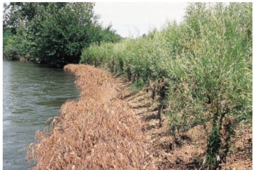
Figure 9.19: Revegetation project, 1 to 2 years postconstruction. At the end of a 2-year period, 50 percent or more of the original plantings should be healthy and growing well. Source: King County, Washington.
