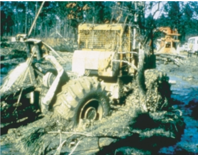
Figure 9.9: Lessons to be learned. Heavy equipment can quickly reduce a vegetated area to churned earth.
