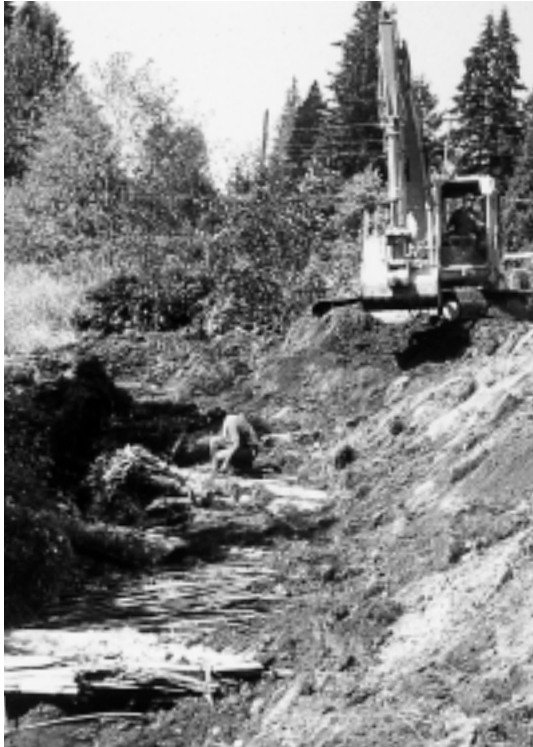
Figure 9.7: Backhoe in operation at a restoration site. Backhoes are mobile in rough terrain and can move rocks and logs with remarkable precision. Source: M. Landin.
