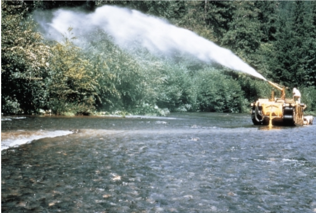
Figure 9.8: Hydroseeding of a streambank. Special tank trucks carrying seed, water, and fertilizer can be used in revegetation efforts.
