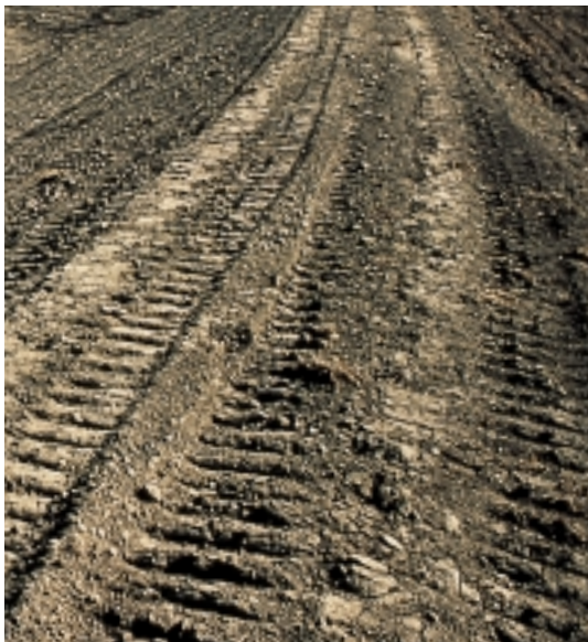
Figure 9.11: Track-roughened area. Rough-textured slopes provide a much better environment for seedlings than do smooth-packed surfaces.
