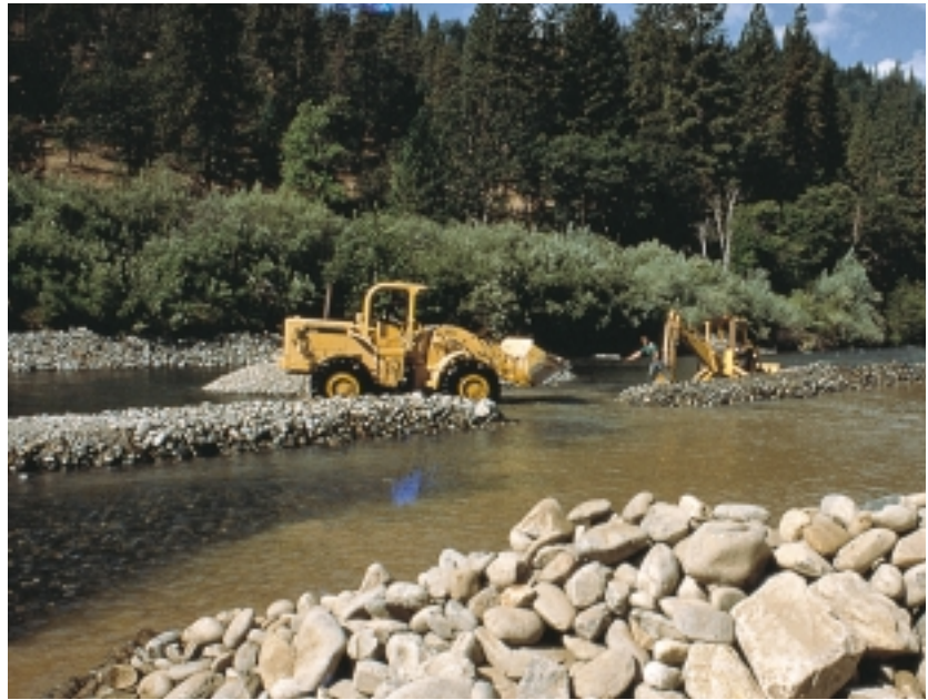
Figure 9.5: Heavy equipment. Avoid heavy equipment in stream channels unless absolutely necessary.
