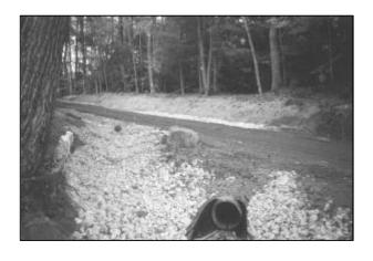
3. To improve the drainage, ditches were constructed on both sides of the road and culverts were used to direct water to stable outlets.
