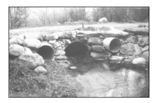
3. Headwalls and endwalls were constructed using stone found on site. The new culverts are expected to adequately handle heavy flows, thereby improving the protection of the road.
