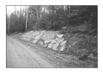
3. A Work in Progress: To stabilize the bank, the town used a combination of small and large rocks on the face of the bank. A ditch was constructed along the toe of the slope and culverts were used to direct runoff to stable outlets before it reached the river.
