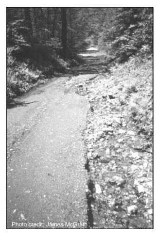
The negative effects of water are clearly illustrated in this photograph. The erosive forces of the flowing water have "blown out" this sloping unpaved road, rendering it virtually impassable.
