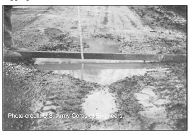
Repair with spot grading (undercut potholes with grader blade—don't just fill them in!)
