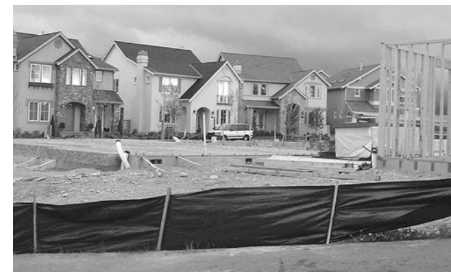
In phased construction, completed portions are permanently stabilized before other areas are disturbed.
