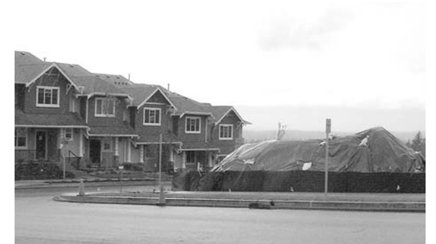
Covering dirt piles reduces storm water runoff velocity.
