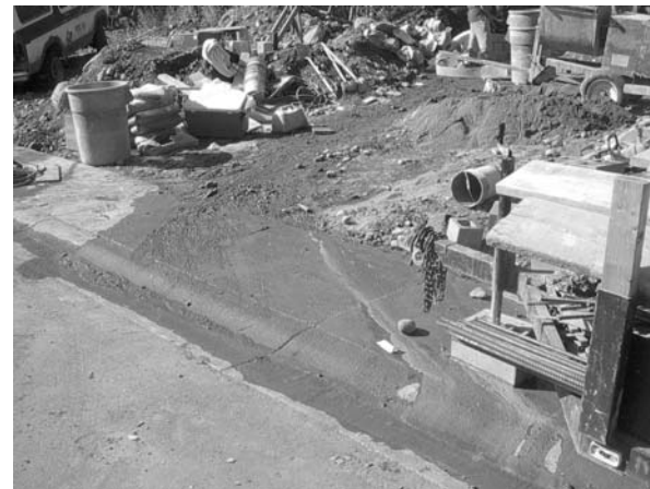
Improper management and disposal of wastes can result in polluted storm water discharges.
