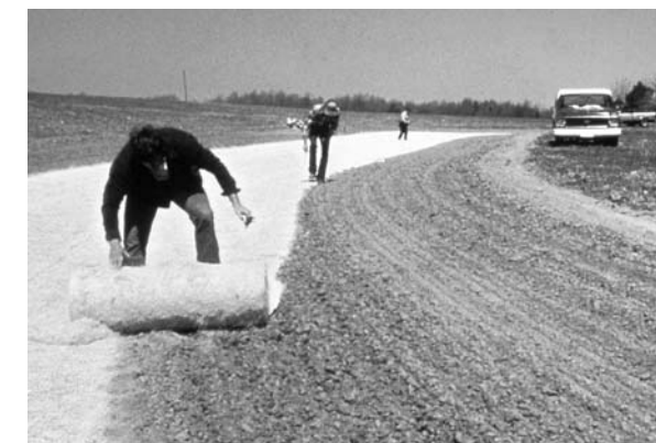
Exposed soils are very vulnerable to erosion. Mulch or other ground cover protects surfaces from wind and storm water erosion, as well as allowing vegetative growth.
