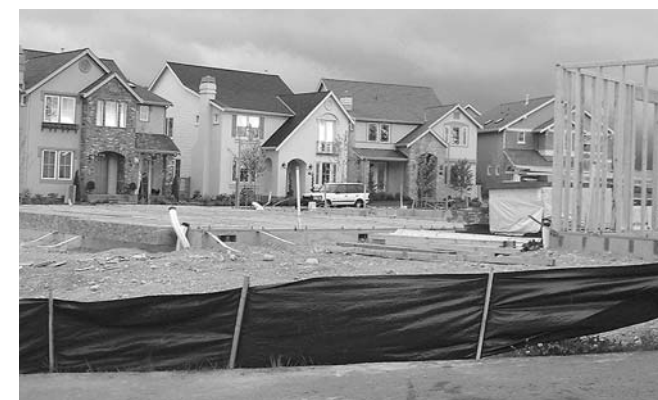
In phased construction, completed portions are permanently stabilized before other areas are disturbed.
