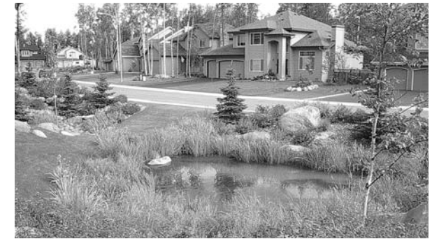
Constructed wetlands can be an effective - and attractive - post-construction storm water control.
