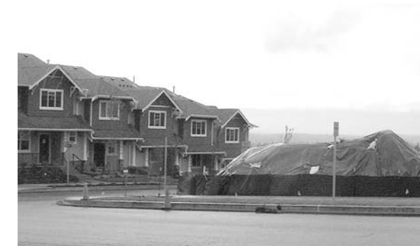
Covering dirt piles reduces storm water runoff velocity.
