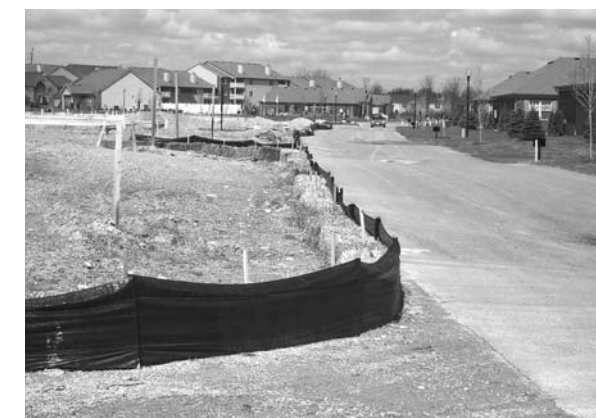
Silt fences prevent the offsite transport of sediment at construction sites.
