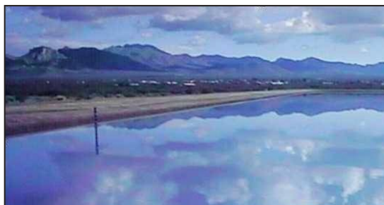
Figure 12 - Clearwater Recharge Facility
