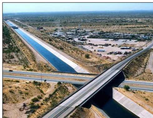
Figure 11- CAP canal east of Phoenix
