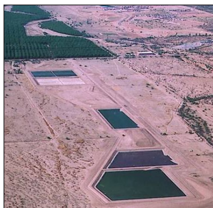
Figure 15 - Pima Mine Road Recharge Project
