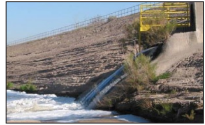
Figure 17 - Treated discharge from treatment plant
