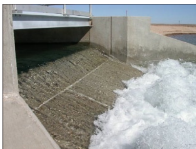
Figure 13 - Water flows into excavated basins
