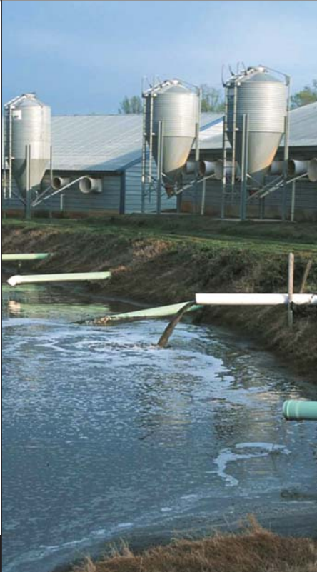
State-of-the-art lagoon waste management system, located in Georgia, for a 900-head hog farm. This facility is completely automated and temperature controlled.
