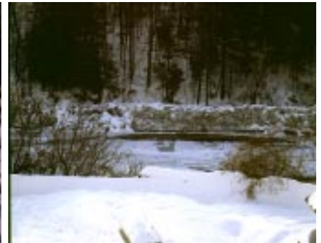
Shear walls (after jam)
