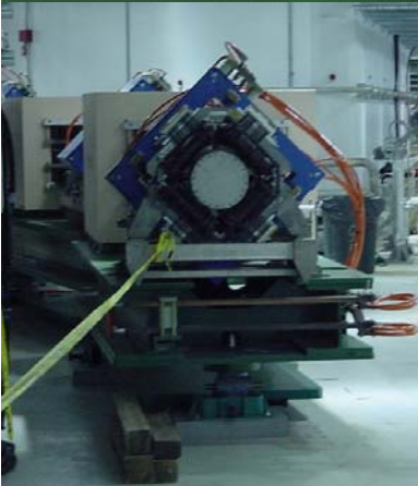
Magnets staged in the HEBT tunnel
