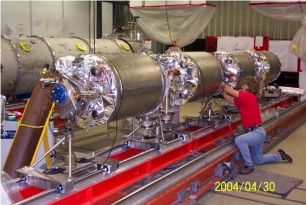
String assembly for cryomodule High- \beta 1
