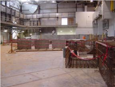
Poured in place shielding for the Backscattering Spectrometer Instrument
