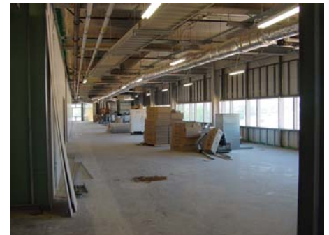
CLO Third floor construction
