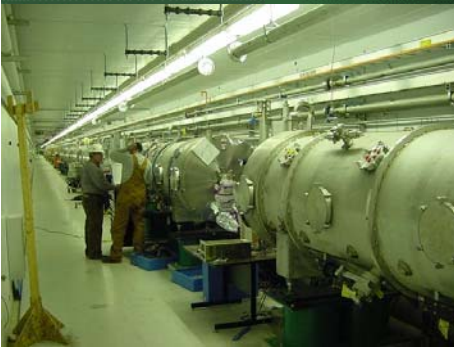
Cryomodule Installation
