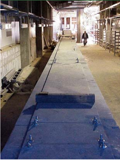
Guide support installation in the 2TU Beamline
