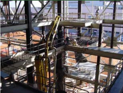
Target Mezzanine construction
