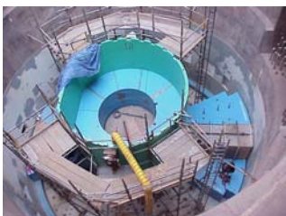
Shielding Block installation
