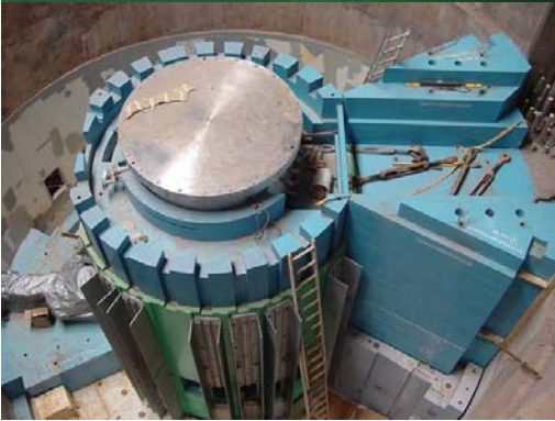
Target monolith showing shielding blocks and inner guide rails
