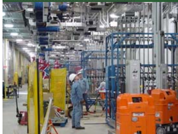
Klystron Building installation
