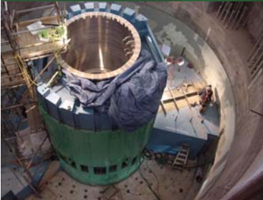
Welding of the chimney to the core vessel
