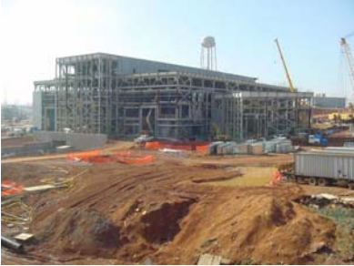
Target Building Construction
