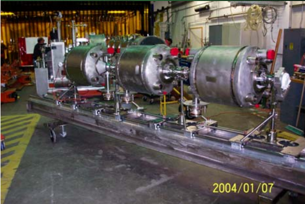
String Assembly for cryomodule M-9
