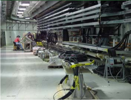
Installation in the Ring Injection section
