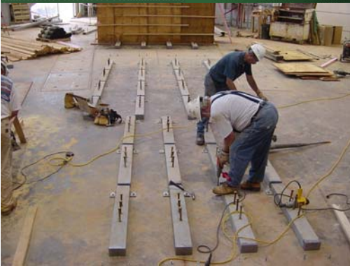
Installation of flight tube supports for the Backscattering spectrometer
