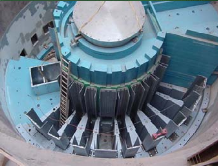
Target monolith showing shielding blocks and inner guide rails
