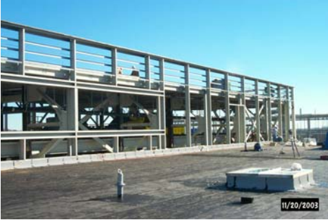
Target Building High Bay steel
