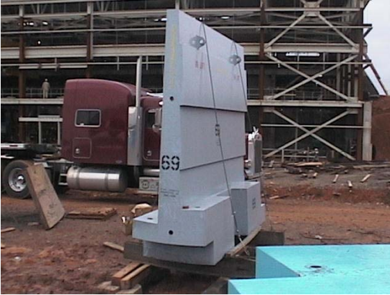
Interstitial shielding blocks on site ready for installation
