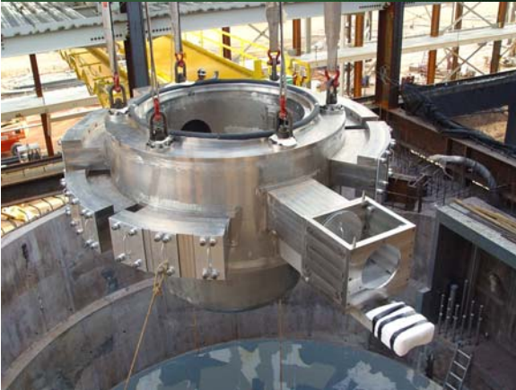
Core Vessel Installation
