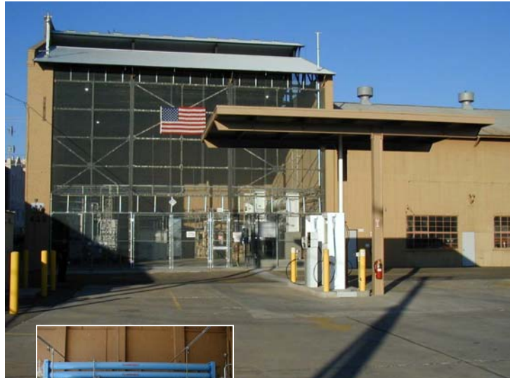
Alternative Fuel Pilot Plant and fueling island (above) and hydrogen low-pressure and two high-pressure storage tanks with PEM electrolyzer (inset at left).
