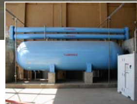
Alternative Fuel Pilot Plant and fueling island (above) and hydrogen low-pressure and two high-pressure storage tanks with PEM electrolyzer (inset at left).
